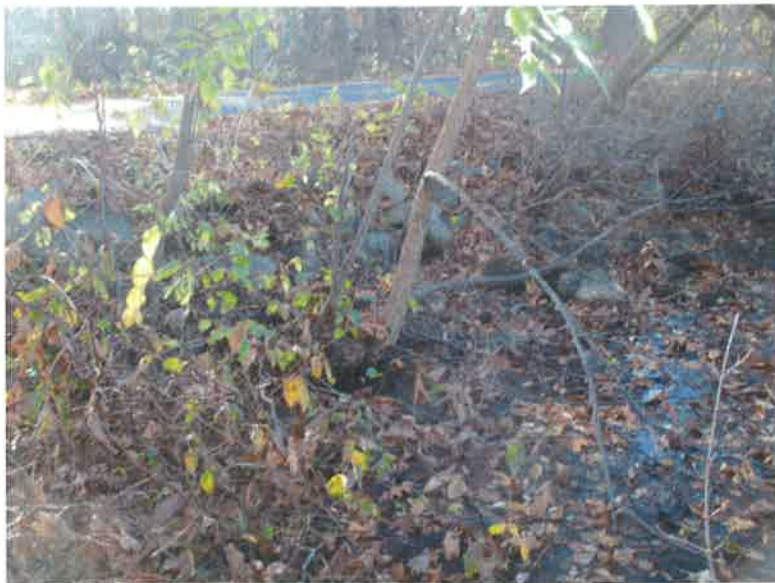
The existing hydraulic crossing of the driveway viewed to the south
