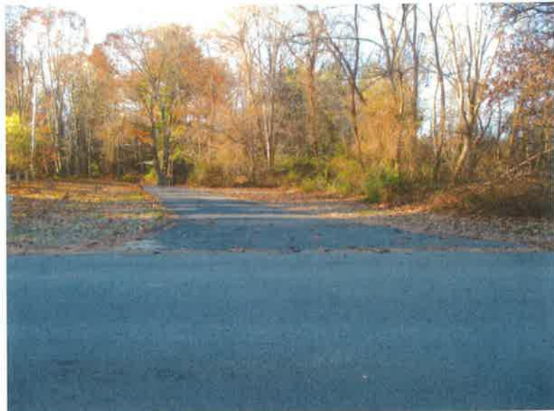
Existing driveway and proposed location of new roadway at Perkins Row.
